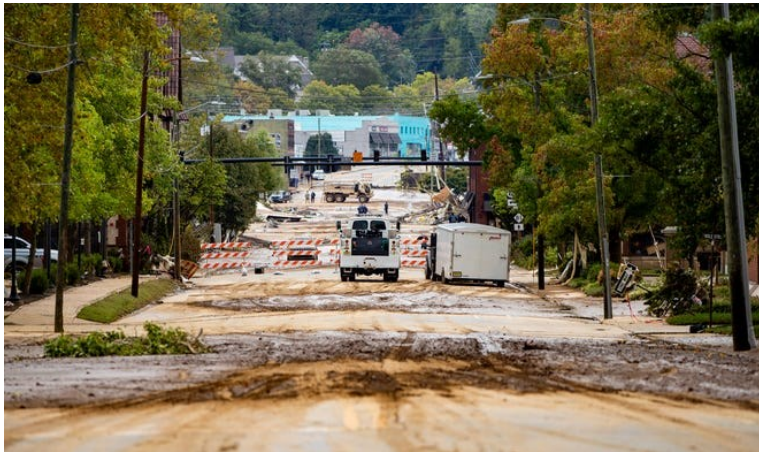
Crews work along Hendersonville Road at the entrance to Historic Biltmore Village Sept 27 in Asheville, NC, after Tropical Storm Helene.—Josh Bell/Asheville Citizen-Times
